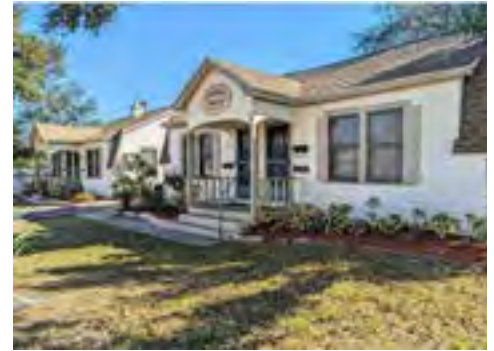
BAYVIEW VILLAS 442 30TH AVE N ST. PETERSBURG, FL
