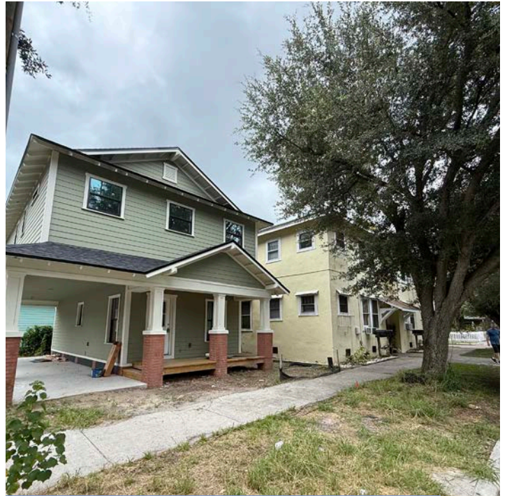
Adjacent SFH Being Built on 0.05 Acres
